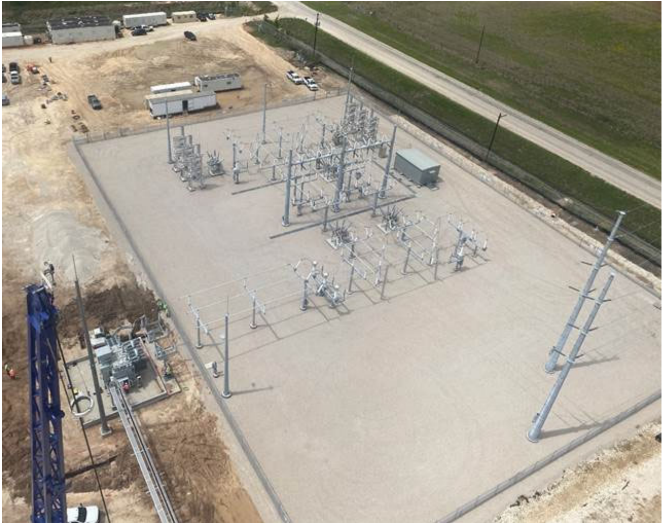
Aerial view of a major portion of the project
