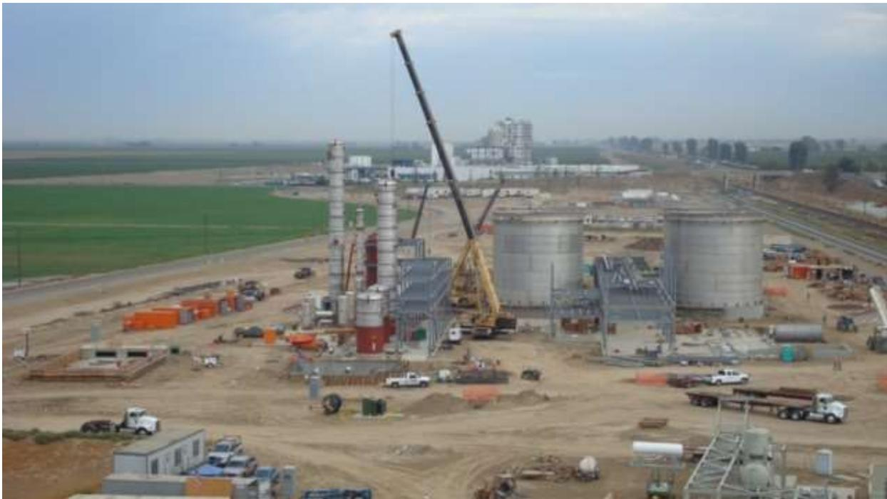
*Pictured is a 50 million gallon per year (MMGPY) fuel ethanol plant in California in early phases of construction. The site was a greenfield host to a cogeneration facility. Based on client measurements and reporting for carbon credits, this is the most energy efficient plant in California and likely all of the US.*
